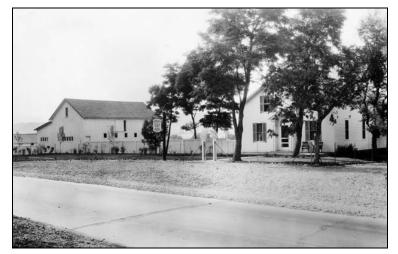
**Figure 30.** The first application of concrete in the state highway system occurred with the 1918 paving of the Great North-South Highway (also US 85, SH 1 and Santa Fe Drive). The initial 16-foot wide strip ran from Littleton to Denver. Photographer: Rocky Mountain Photo Company, August 6, 1924. Source: Denver Public Library, Western History Department.
