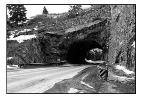
**Figure 47.** The Ouray Tunnel on US 550 dates to the early 1920s when, after a major construction project, the former toll road emerged as the "Million Dollar Highway." The tunnel was widened in 1958. The granite outcropping did not require a supporting portal structure. A dry-laid stone wall over the tunnel entrance holds the slope and diverts run-off. Source: ACRE, 2002:11-7.
