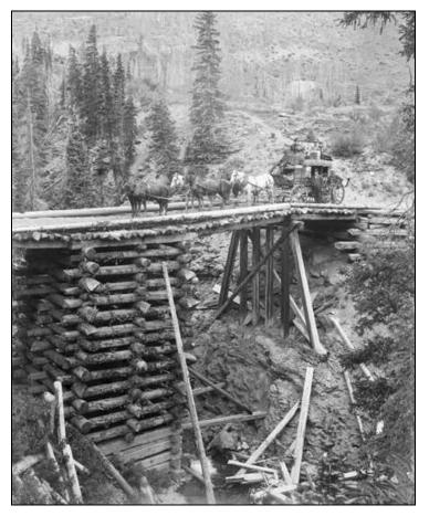
**Figure 4.** A three-team stagecoach crosses an impressive timber pile bridge in western Colorado near the end of the nineteenth century. Photographer: Harry H. Buckwalter. Source: Colorado Historical Society
