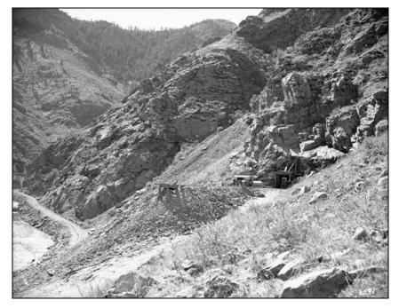
**Figure 19.** Work progresses on a highway tunnel in Clear Creek Canyon in the late 1940s. Tunnels straightened highway alignments allowing motorists to travel at higher speeds. The original road around the outcropping is visible to the left. Photographer: Bob Zeller. Source: Colorado Historical Society.
