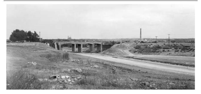
**Figure 20.** A pair of bridges stands partially completed in 1949. Though begun before the initiation of the Interstate highway program, the Valley Highway in Denver benefited financially by being absorbed into the new federally funded construction program. Source: Denver Public Library, Western History Department.
