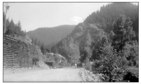
**Figure 35.** Mine and mill operators used wood crib walls to stabilize steep slopes. The technology readily transferred to highway construction. Photographer: Muriel Sibell Wolle, 1955. Source: Denver Public Library, Western History Department.
