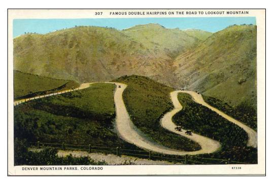
Figure 10. The Lariat Trail winds its way up Lookout Mountain above Golden. Designed for automobile touring as part of the Denver Mountain Park system, this early postcard shows the route's double hairpin curves. At one point the trail was part of the nationwide Victory Highway. Source: Office of Archaeology and Historic Preservation, Colorado Historical Society.
