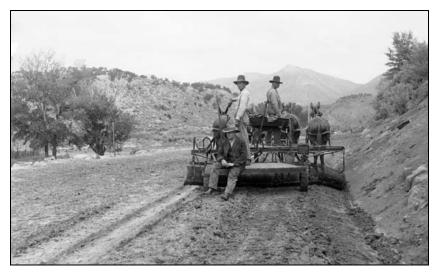
Figure 27. A road crew grades a highway in western Colorado. Dirt roads required constant maintenance to deal with the ravages of traffic and weather. Photographer: Either Fred Garrison or Ola Aftinson Garrison, June 5, 1924. Source: Colorado Historical Society.
