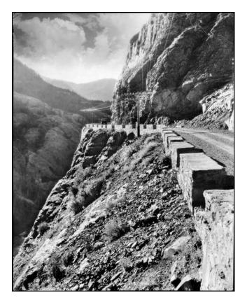
**Figure 13.** Otto Mears' Red Mountain toll road had a much safer appearance in the late-1920s than in its wagon road days (*Fig. 6*). In addition to providing protection for motorists, the crenellated stone shoulder guard added to the aesthetic qualities of this scenic mountain highway. Source: Denver Public Library, Western History Department.
