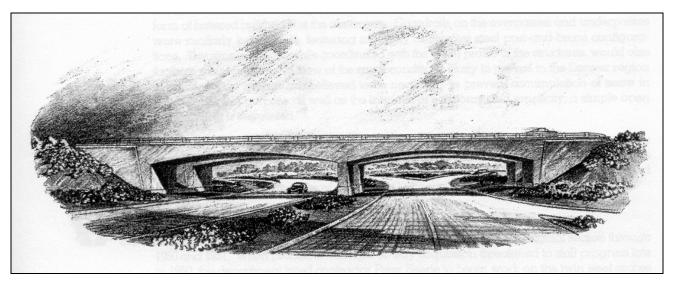
**Figure 65.** The overpasses designed in 1944 for the Valley Highway typically consisted of paired identical structures. The bridges employed an architectural formality that was as much aesthetic as practical. Designers Crocker and Ryan described their design as "devoid of special architectural organization or ornament, in the belief that the simplicity of such construction and its direct expression of function will have full aesthetic value." Source: Hermsen Consultants, 2000: 23-24.
