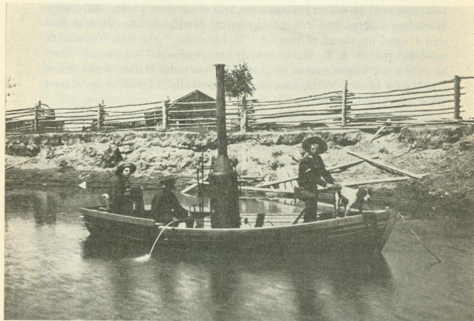
FIRST STEAMBOAT ON UPPER RIO GRANDE, AT ALAMOSA Gov. Hunt's sons equipped their boat with a small upright steam boiler and engine. In the boat are (left to right): unknown, Bert Hunt, Bruce Hunt.
