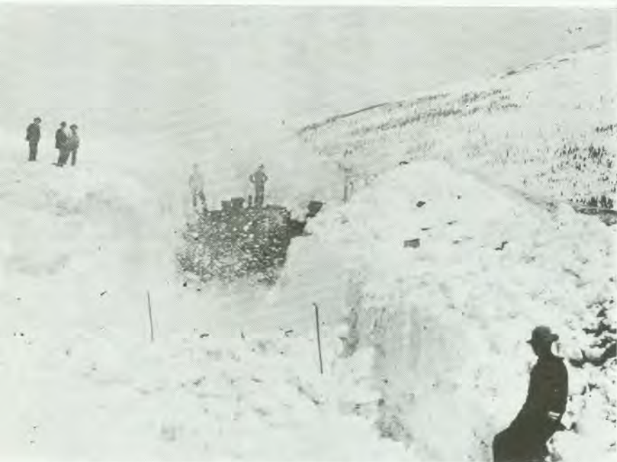
10200's cutting wheel hurled snow and rocks from the tracks. The original blades were soon chewed up and replaced with special "V" blades.
