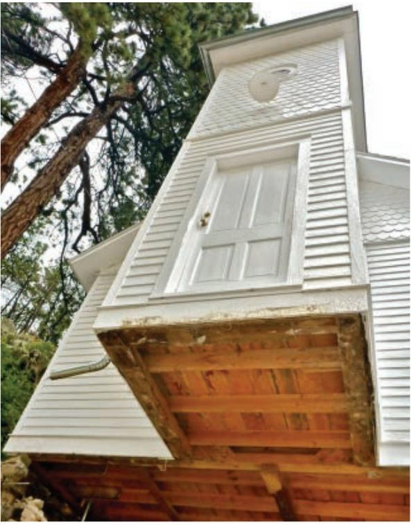
*This page and facing: State Historical Fund emergency dollars enabled stabilization of Salina's historic Little Church in the Pines after floodwaters ripped away half the foundation.*
