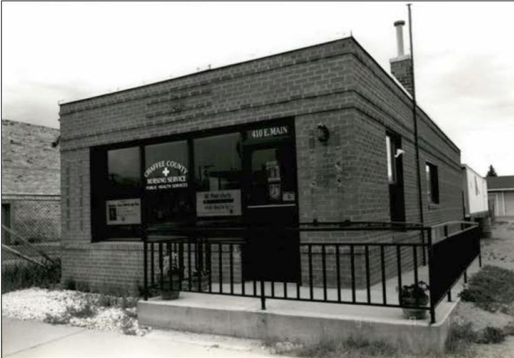
Figure 5. The Chaffee County Nursing Service still occupied the building in 1994. The building had received replacement door and windows (three fixed windows instead of four on the front) and a pedestrian ramp by that time. SOURCE: Hartley and Schneck, survey photograph July 17, 1994.
