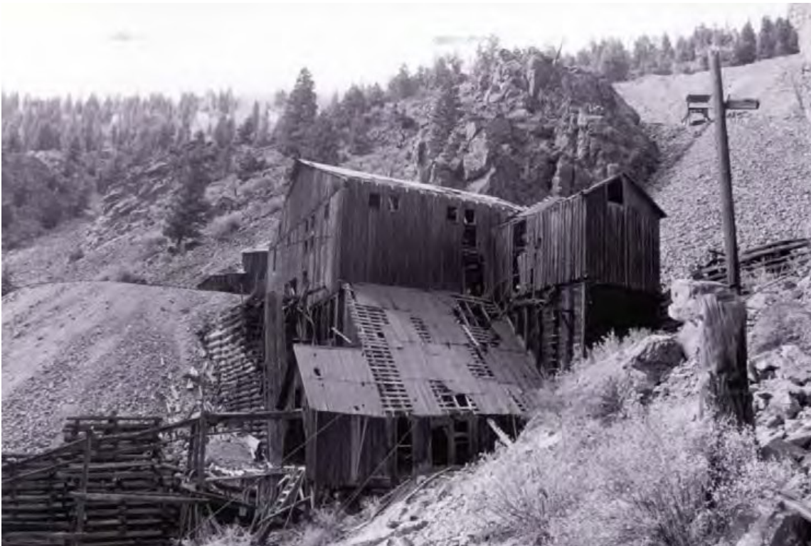
Historic Photo 11. Lower Bachelor Ore Sorting House with Aerial Tramway Terminal, 1999; camera facing southwest. Photo by Eric Twitty from Mining the Amethyst Vein , Vol. 1, 79.
