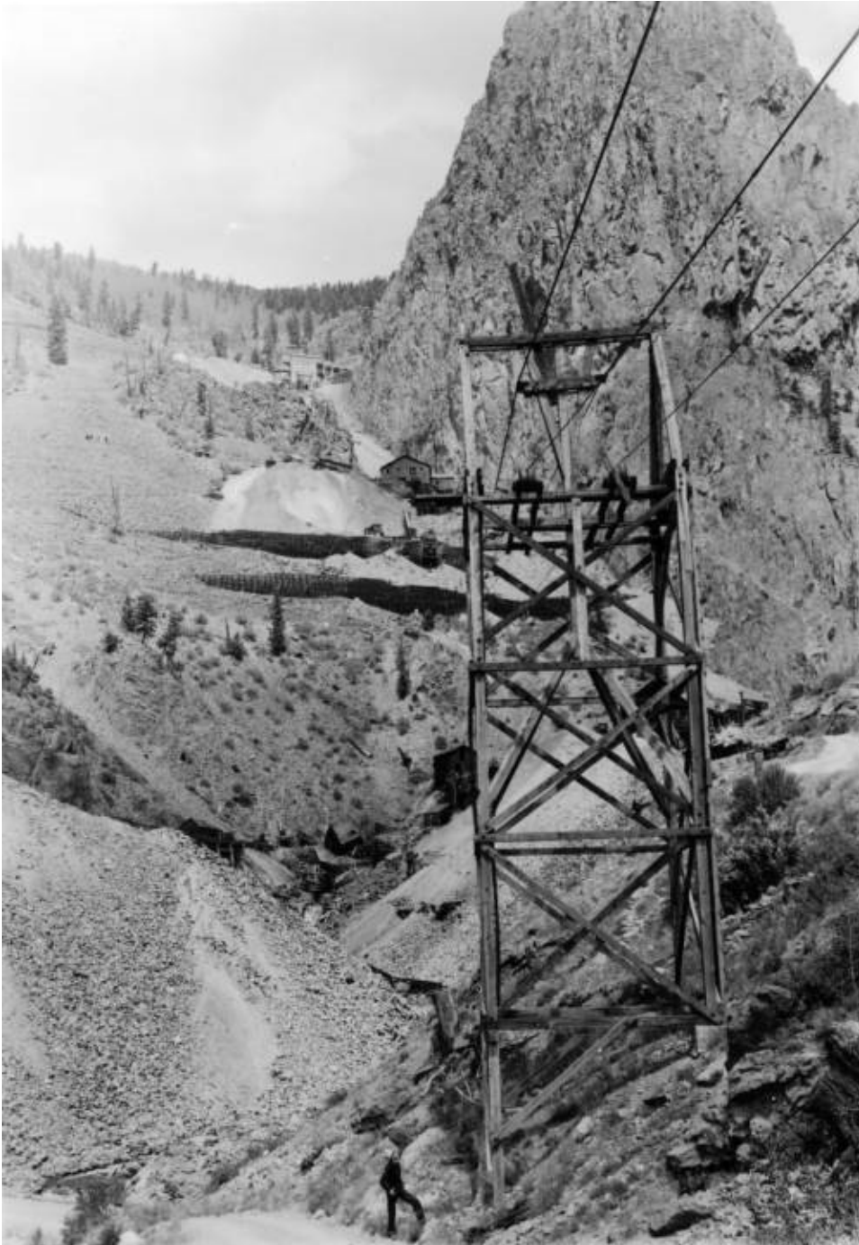
Historic Photo 4. Photograph (1942) showing Bleichert double-rope aerial tramway tower (not extant) in foreground. The Commodore Tunnel is visible through the tower. The Lower Bachelor complex is above, its dump retained by two log cribbing walls. The prominent gabled building perched on the dump is the tramway's ore sorting house and upper terminal. West Willow Creek cascades through the foreground. The large waste rock dump at left belongs to the Nelson Tunnel (not extant and outside of the Bachelor-Commodore boundaries). Photograph by Theodore Fisher. Photo courtesy of Denver Public Library Special Collections, call number X-61937.
